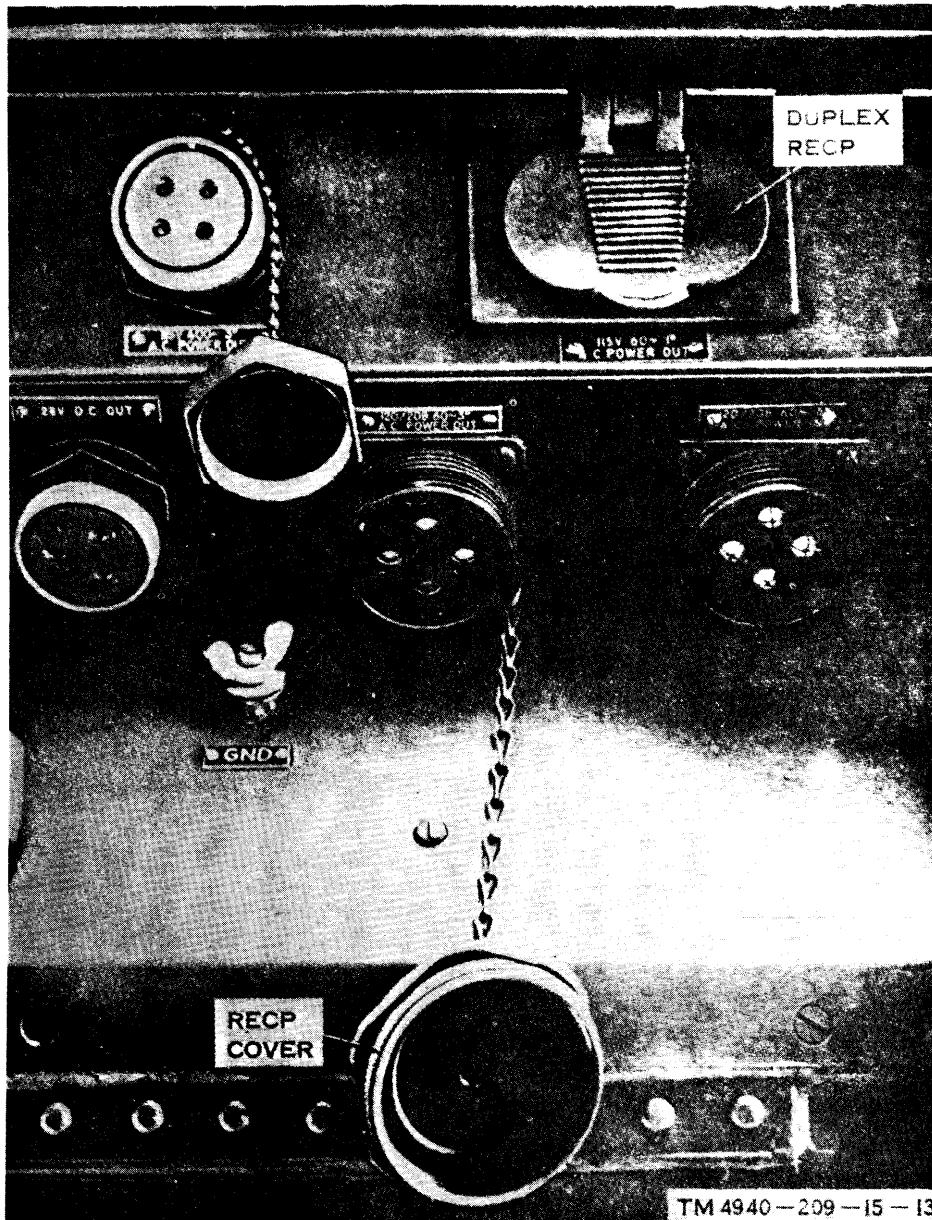
Figure 1-4. Repair van, power entrance box.
